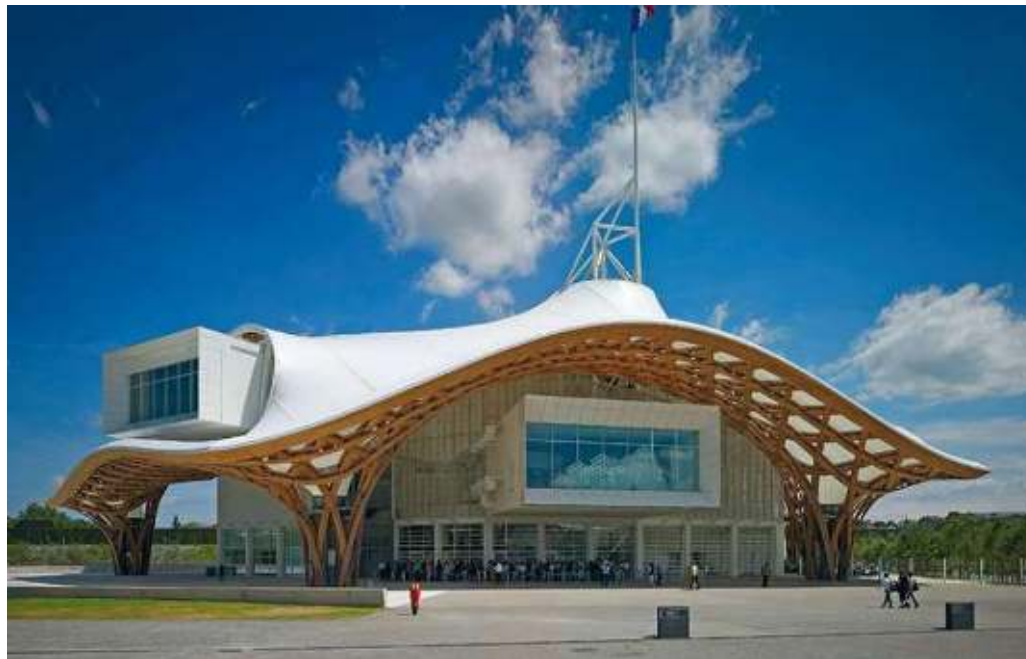
Centre Pompidou Metz
